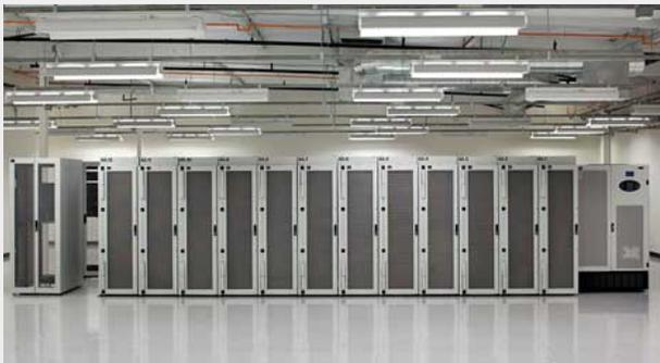
A row of cabinets inside the Colovore data center in Santa Clara, Calif. Each cabinet is equipped with a rear-door heat exchanger using tempered water.
